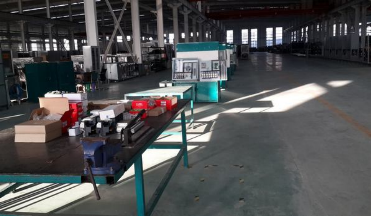
Electric Control Workshop
